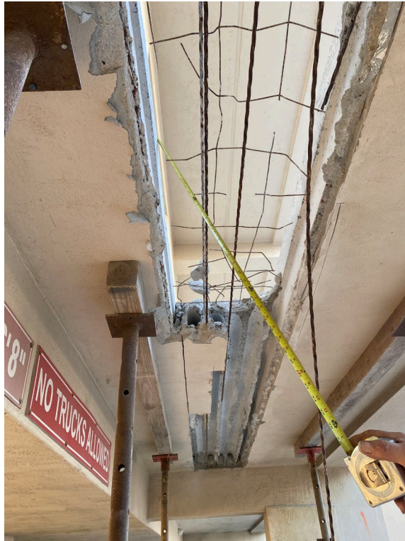
Picture 3: In-progress walkway repair
