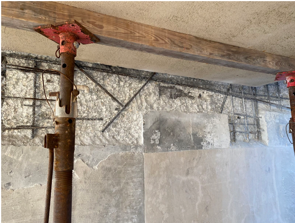
Picture 2: Completed excavation prior to steel cleaning
